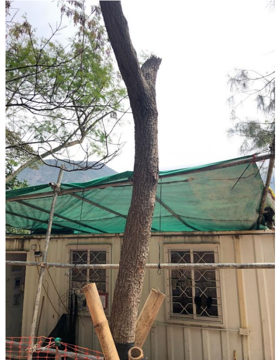
Photo 17: Trunk condition of G62/RT-07
